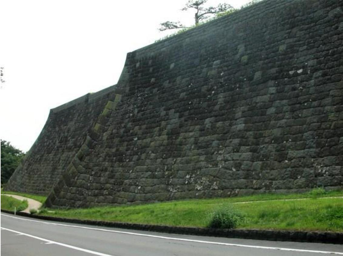
The dark-coloured stones are original; lighter-coloured stones are new stones replacing original stones which were too damaged to be reused in the reconstruction of the walls.
