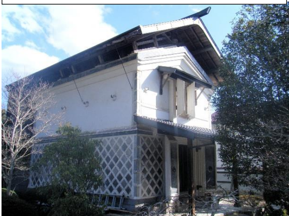
Fig. 15 Warehouse before the disasters (March 7, 2009)
